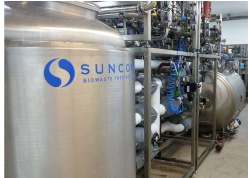
HybridEDS™ with separate tanks for Collection and Treatment
